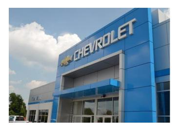
11. Metal Paneling with concealed fasteners (May not exceed 30% of a total area of any one façade)
