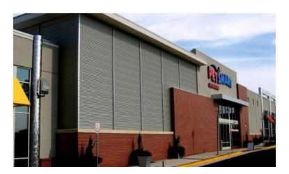
12. Metal Siding with a sine wave pattern (May not exceed 30% of total area of any one façade)
